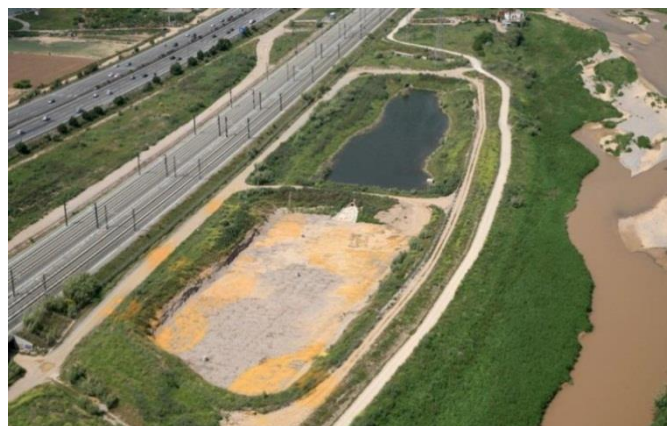
Figure 3-15: Aerial picture of groundwater recharge system at Sant Vicenç dels Horts
